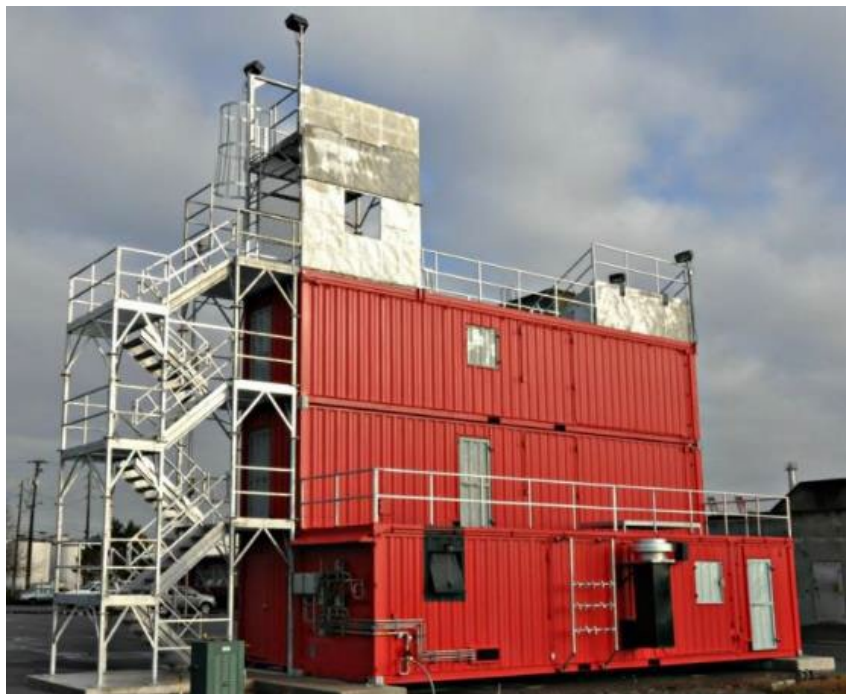
Live-Fire Training Prop – Training Center
